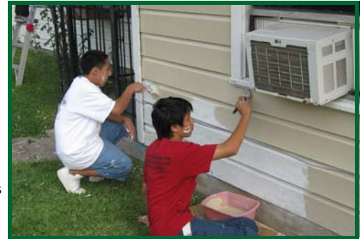
KIPP high school students repaint a house damaged in Hurricane Ike.
